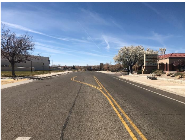
Figure 20: Homestead Cir. facing west at Taylor Ranch Rd.
