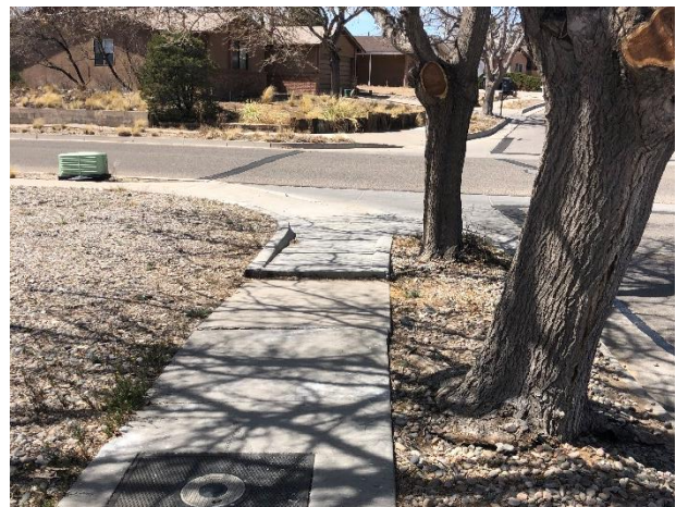
Figure 13: Sidewalk on Kettle Rd. at Mojave St.
