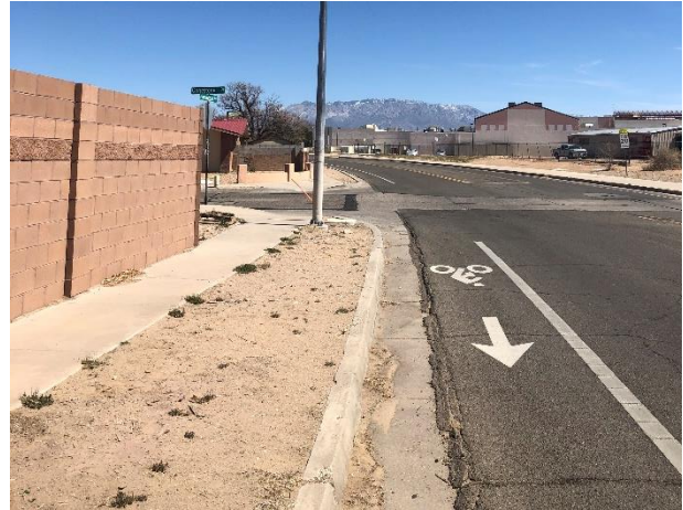
Figure 23: Sidewalk on Homestead Cir. at Conestoga Dr.
